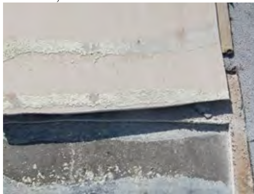
Fig.4 Soft, off ratio foam adhesive coming apart; cohesive failure within the foam
